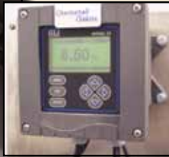
Automated Chemical Test Pretreatment chemicals are monitored and added automatically but titration is checked manually twice per shift.
