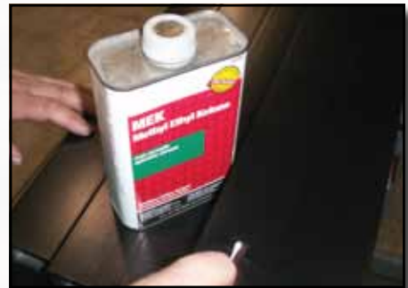
PCI#8 Solvent Cure Test Solvent testing per PCI#8 is completed hourly to test for complete cure.
